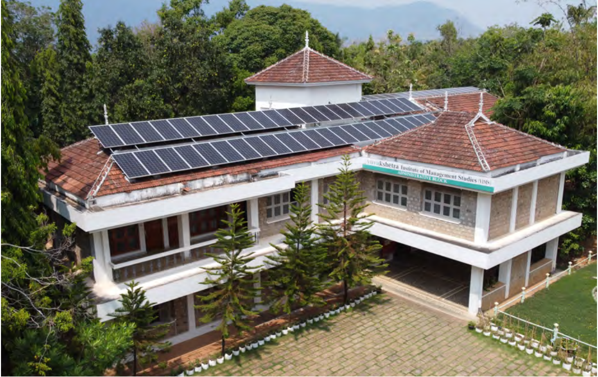
35 kW SPV Installation on rooftop of YIMS Administrative Block
