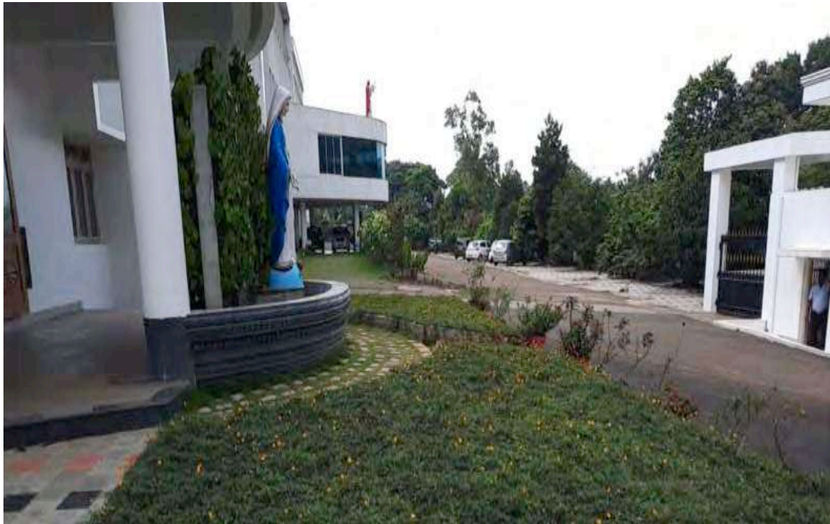
Landscaping in progress in own campus
