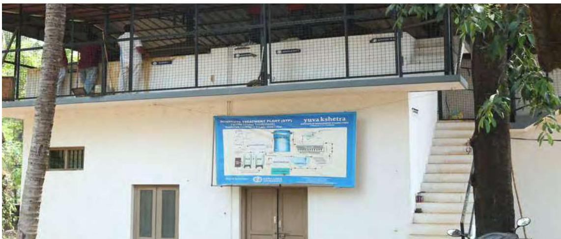
Water Treatment Plant at YIMS
