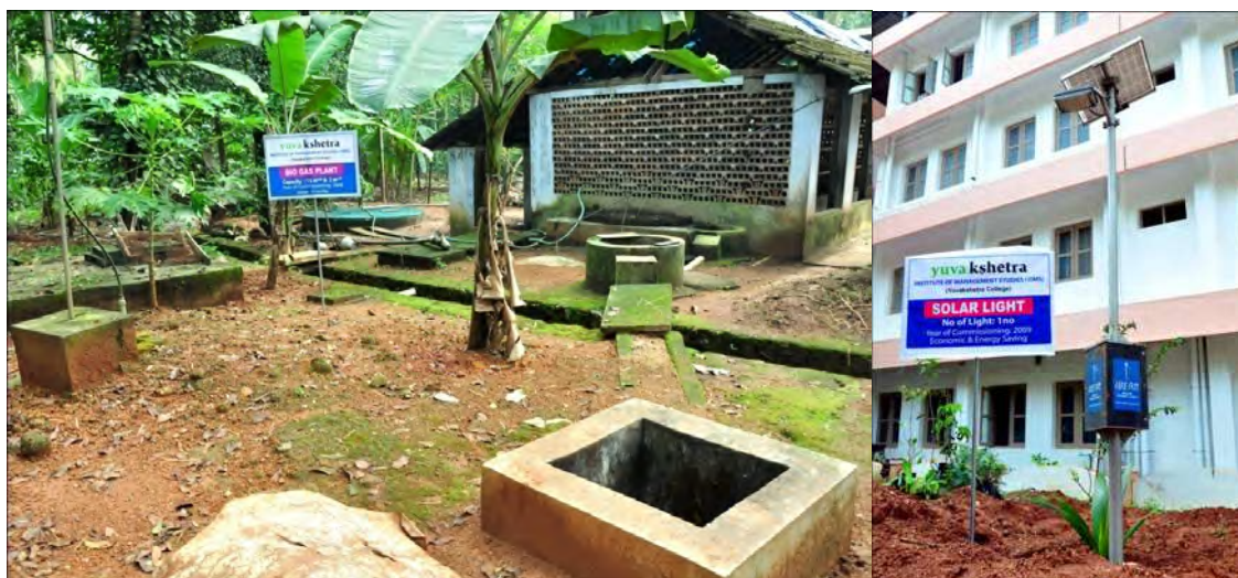
Biogas plant at YIMS (left); (Right) Solar Street light installed in 2009
