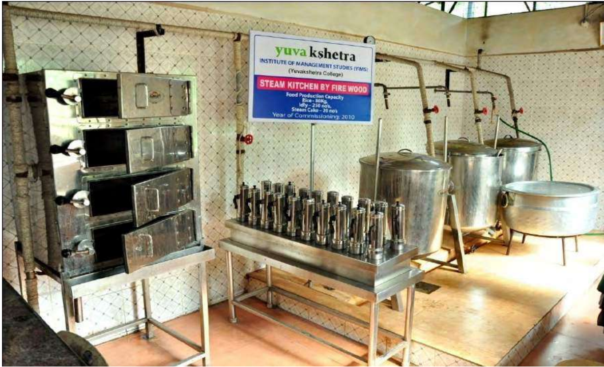
Steam Cooking room at YIMS Can cook 80 kg of rice/250 Idlis/20 Steam Cakes ( Puttu ) in one round
